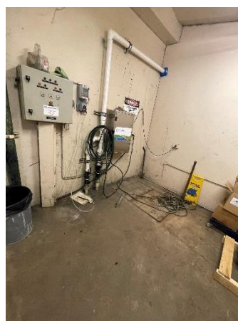
Existing sewer pump station.
